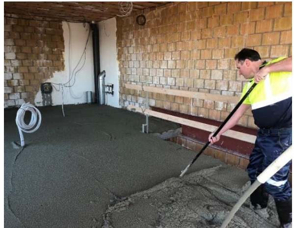
Figure 3: baseTherm® pumping and levelling
