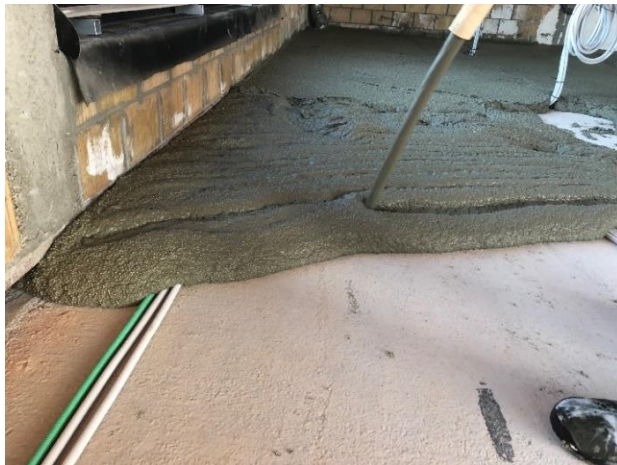
Figure 3: baseTherm® pumping and levelling
